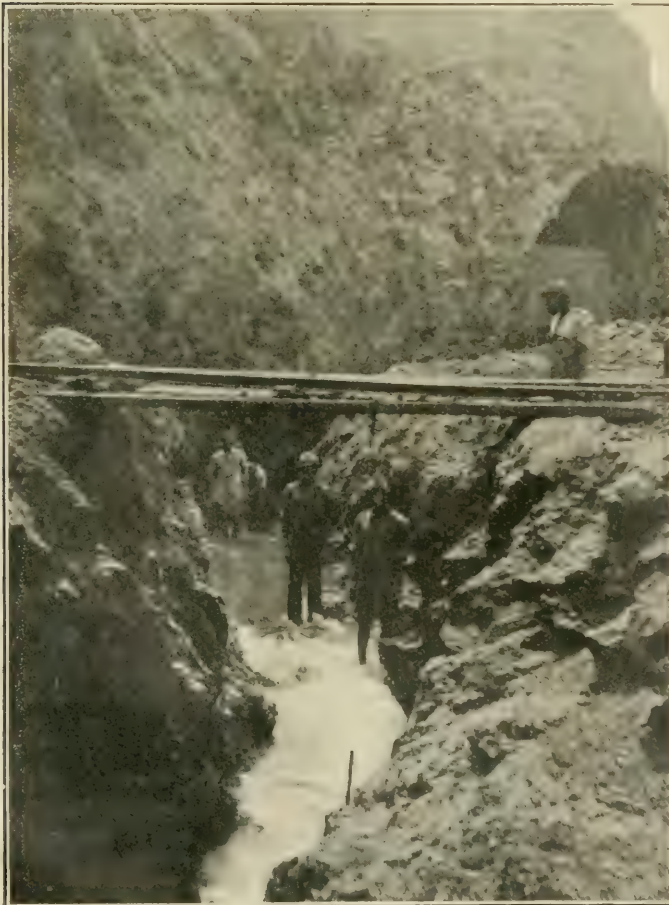
VIEW OF DRAIN AT N.W. CORNER OF OPEN-CUT.
